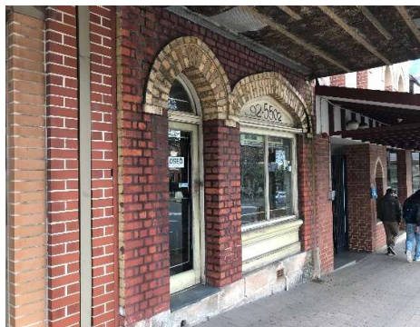
Figure 34 - Shopfront façade showing the two colour brickwork, pointed arches, sandstone base and timber shopfront.
