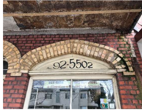
Figure 37 - The pointed arch over the timber framed shopfront window. The transom, framing and infill panel appear to be original.
